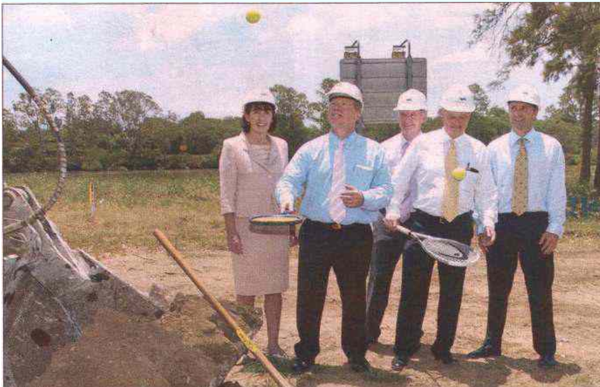
■ A new ball game ... Premier Peter Beattie at the site of the new tennis centre at Tennyson
