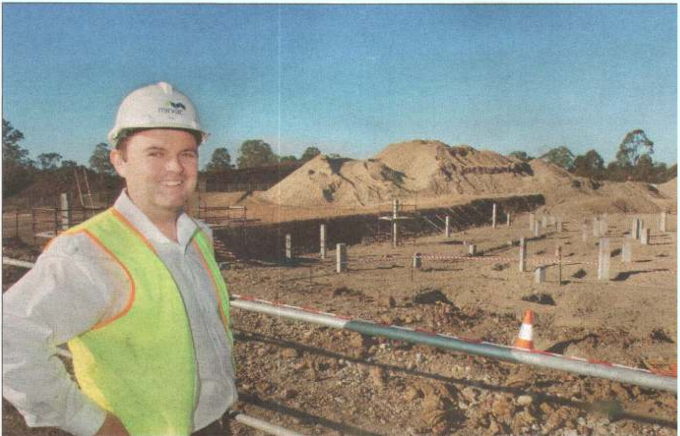
■ Forming foundations ... Tennyson State Tennis Centre project manager Paul Cunningham
